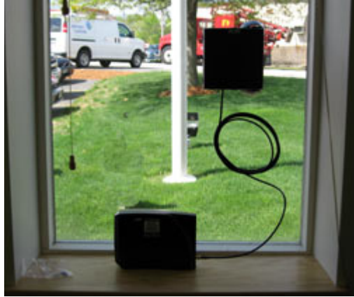
The receiver is attached to the window facing SouthWest with suction cups.
